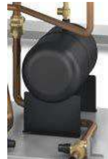
Air cooled condenser tank.
